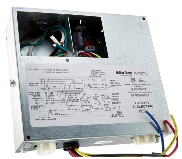
Typical Air Conditioner electronic control module located underneath each of the roof mounted air conditioner coverers. These units always have 12 volts DC supplied to them when either battery switch is on or you are connected to shore power.. If 12 Volts DC is not present at the BLACK/RED 12V lead connections your thermostat or In Command system WILL NOT be able to turn on any of the HVAC (heating and Air) functions
