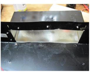
If there are any gaps, cover them with HVAC tape. Reinstall fan housing to the vent hood. Reconnect power wires and then reinstall hood pushing ductwork into vent housing.
