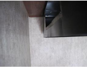
I used a combination square to mark the corners and then drew the outline of the opening. I then used a utility knife with a new blade and cut out the opening. If you are still not sure if a stud is present, run the utility knife along the top part of the cut out. If you hit a stud, stop. Worse case...you have a cut in the wall that will most likely not be visible when you reinstall the hood and fan. Once cut through, carefully remove inside wall piece.
