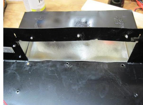
If there are any gaps, cover them with HVAC tape. Reinstall fan housing to the vent hood. Reconnect power wires and then reinstall hood pushing ductwork into vent housing.
