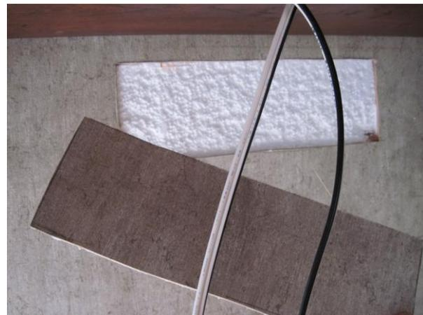
Use the utility knife and a putty knife and remove the Styrofoam. It is not very dense comes out with little effort. It is messy though.
