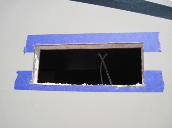
Test fit the vent and enlarge hole if necessary. Also test fit duct piece.
