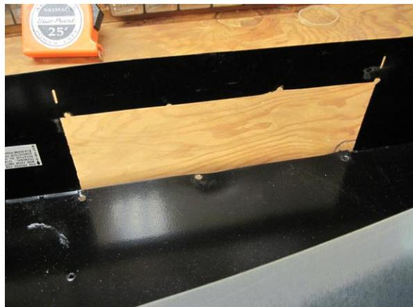
If one side of the hood was mounted directly against a wall you can simply slide it back to the wall and mark the wall using the opening as a guide. If not, reinstall the hood.
