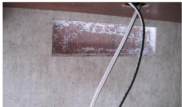
With the hood installed, measure the distance from the back of the hood to the wall and cut a 3.25" X 10" rectangular duct that length. Test fit the duct to make sure everything is lined up correctly. With a small bit, drill a hole through to the outside in each corner of the cut out. Outside the camper put masking tape over the outline to help prevent jagged edges when cutting out the opening. Now cut out the opening from the exterior side.
