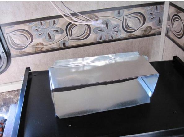
Once you are certain all parts are ready for installation, line the vent edges with butyl tape. Place the vent in the opening and secure with stainless steel screws. Carefully trim excess butyl with a hobby knife. I later sealed vent with RV sealant.
