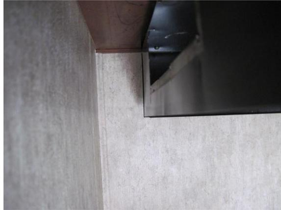
I used a combination square to mark the corners and then drew the outline of the opening. I then used a utility knife with a new blade and cut out the opening. If you are still not sure if a stud is present, run the utility knife along the top part of the cut out. If you hit a stud, stop. Worst case...you have a cut in the wall that will most likely not be visible when you reinstall the hood and fan. Once cut through, carefully remove inside wall piece.
